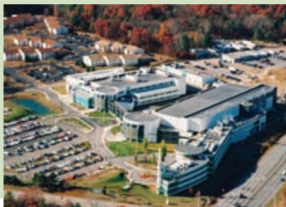
Albany NanoTech Facility
